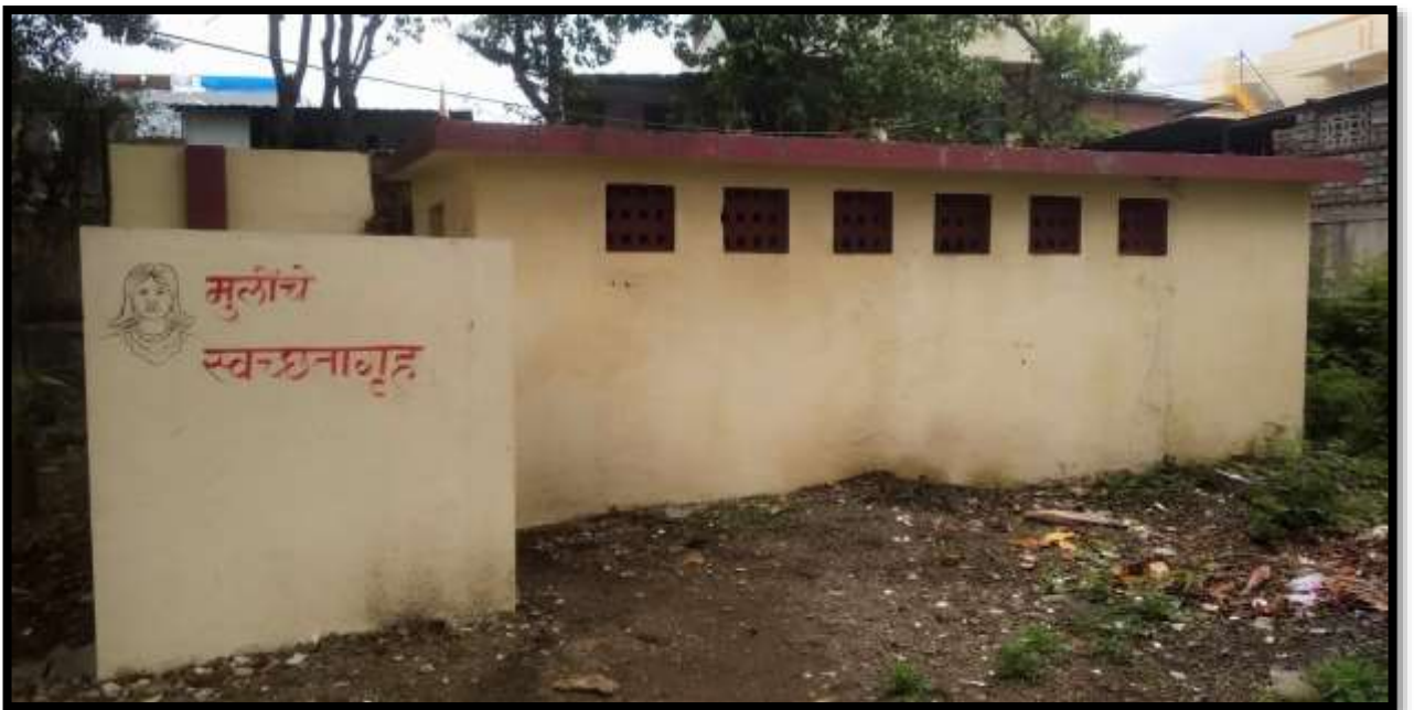
Photo No. 7 Separate Toilet Facility
